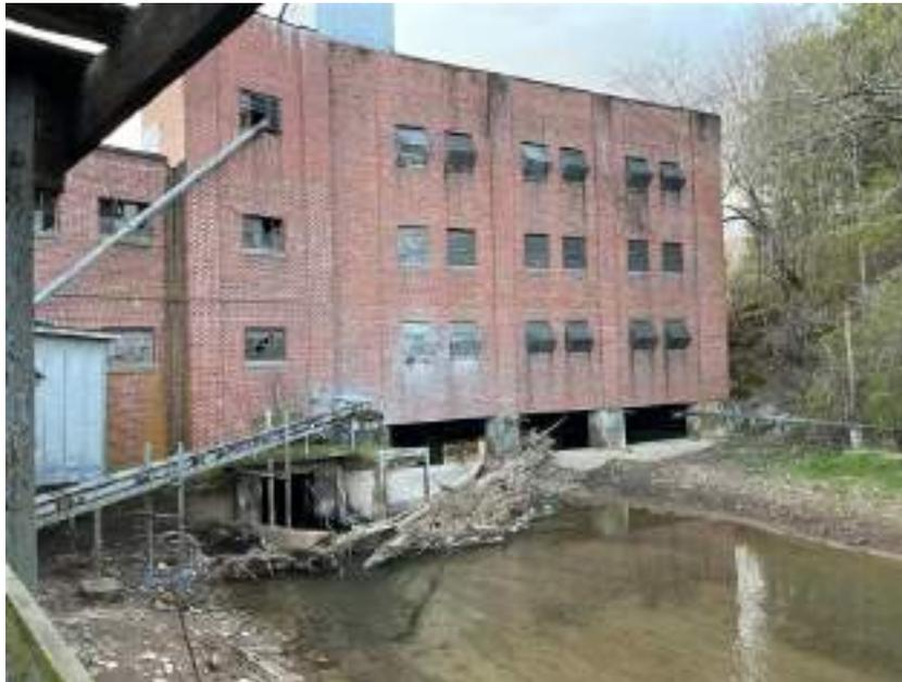
Figure 76: Example of debris captured on dam in North Tazewell
