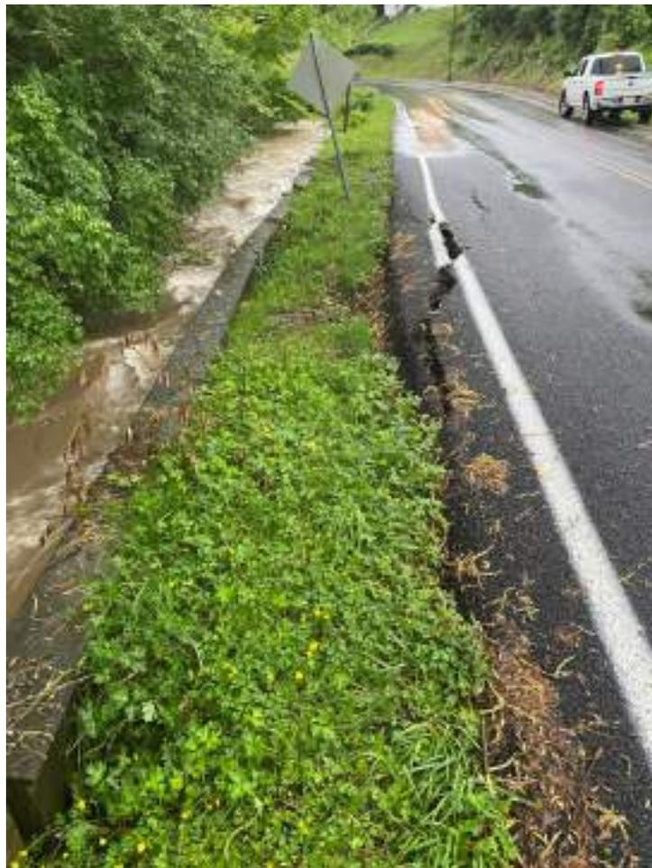
Figure 645: Road Damage in Bluefield, VA from Flooding in March 2023
